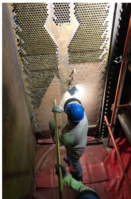
Fig. 4 Inspection of the existing main condenser tubesheet at the Embalse Nuclear Power Plant, carried out in preparation for retubing. Photograph: Nucleoeléctrica Argentina S.A.
